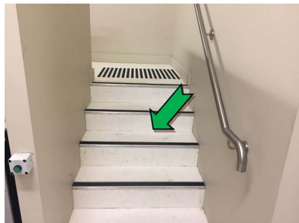
Photo 6. Interior, level one, hall adjacent audio/visual room, floor coverings – suspected non asbestos-containing sheet vinyl.
