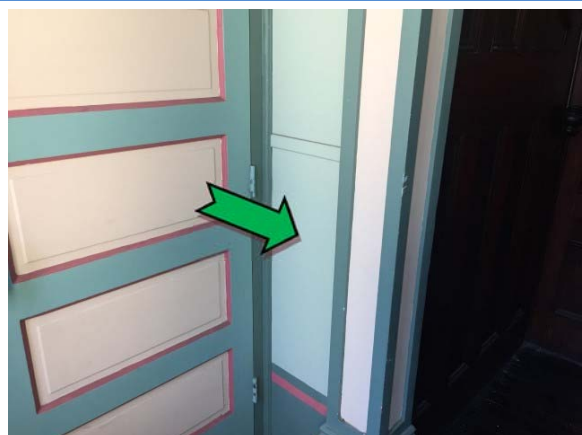
Photo 12. Interior, ground level, north-east elevation, wall – assumed non asbestos-containing fibre cement sheeting.
