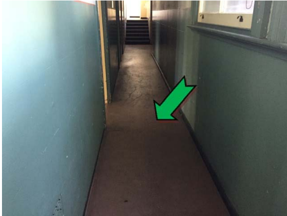
Photo 7. Interior, level one, west corridor, floor coverings – non asbestos-containing sheet vinyl.
