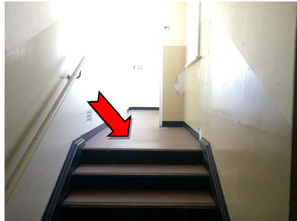
Photo 4. Interior, level one, floor coverings – assumed asbestos-containing sheet vinyl.
