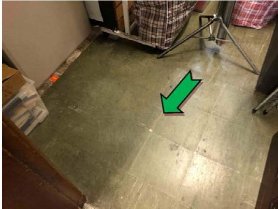
Photo 13. Interior, ground level, floor coverings – non asbestos-containing vinyl floor tiles.
