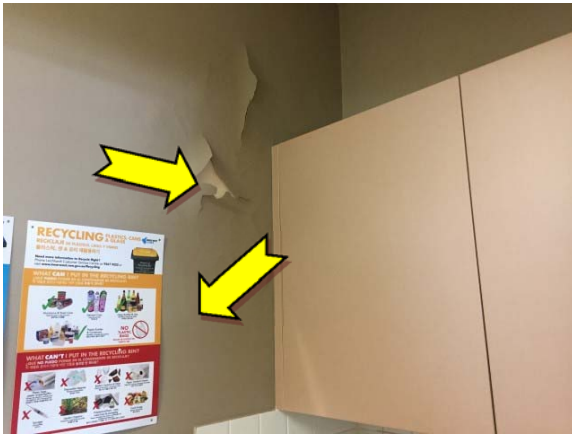
Photo 21. Interior, ground level, throughout, walls – lead-containing white lower and suspected lead-containing green upper coloured paint systems.
