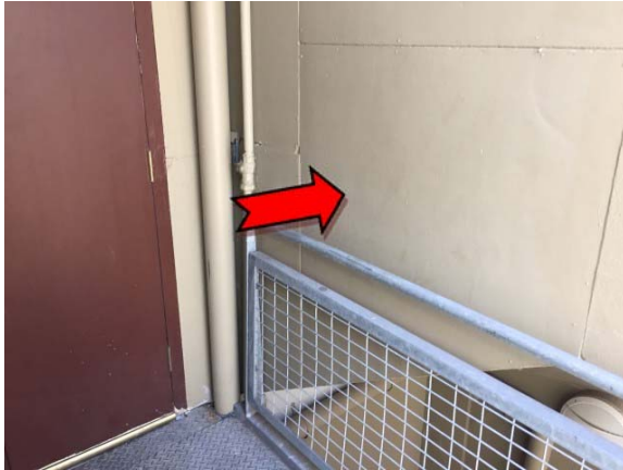
Photo 1. Exterior, level one, fire escape, wall – asbestos-containing fibre cement sheeting.
