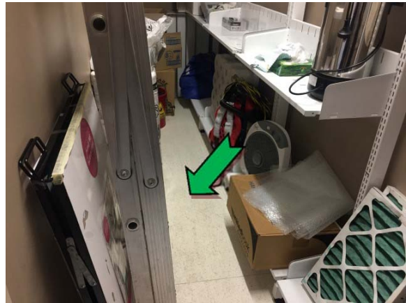
Photo 10. Interior, ground level, meeting room, storage, floor coverings – suspected non asbestos-containing sheet vinyl.
